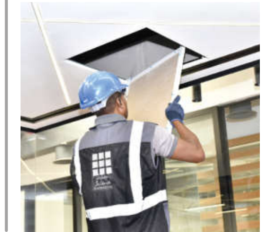
Plain Gypsum Ceiling
