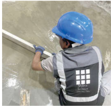
Floor Levelling / Cementing
