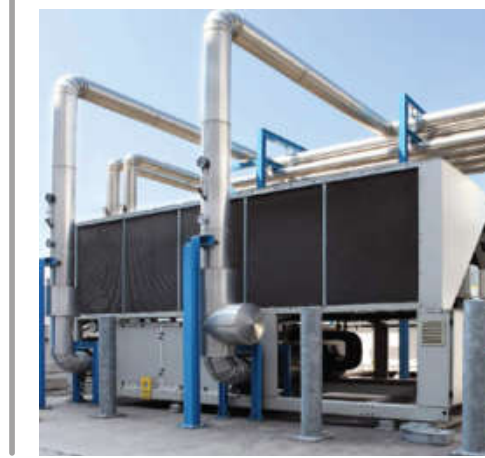
AHU's, FAHU's & VAV's
