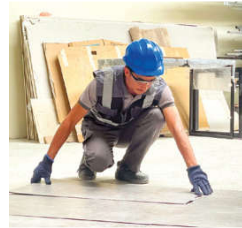
Floor and Wall Tiling
